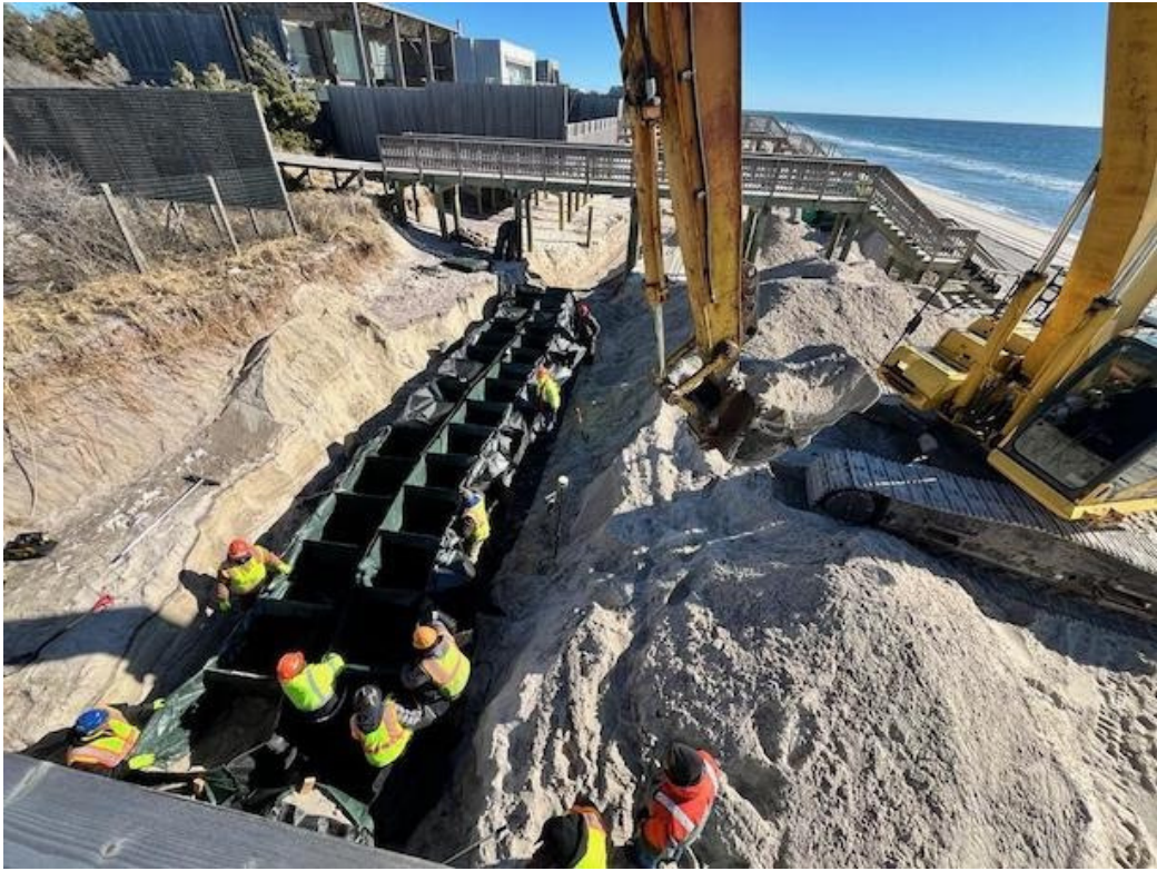
Trap bag installation in the Pines (Photo P. Priolo)
