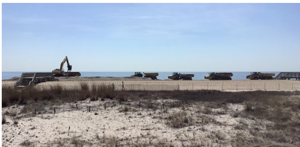
Large trucks drove the sand down to the eastern beaches (Photo Don Sussman)
