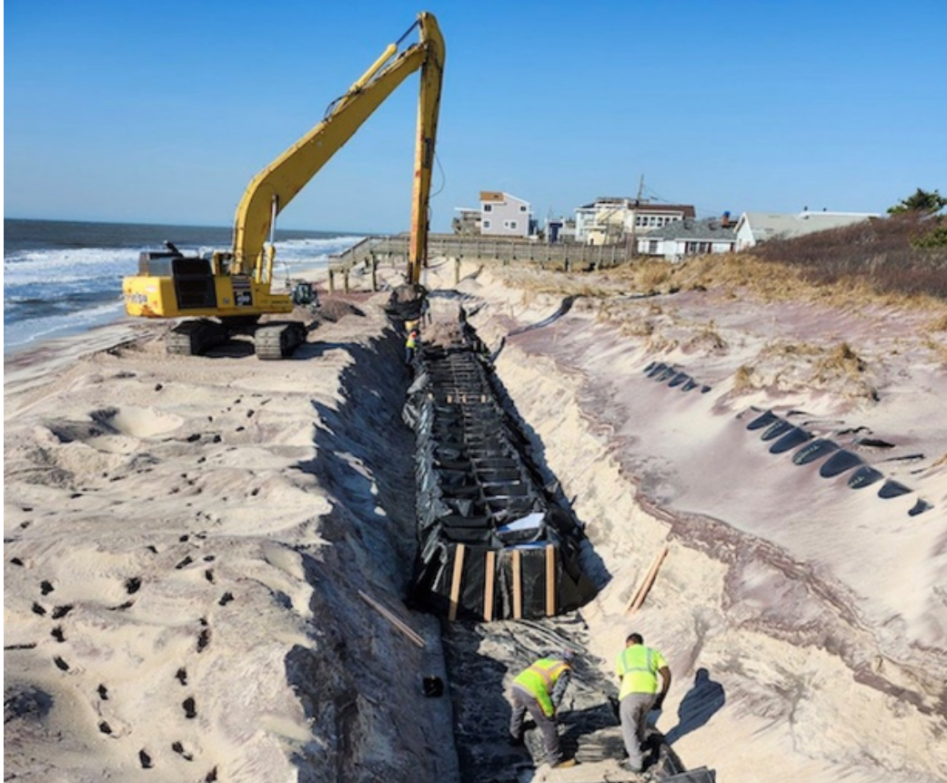
Trap bag installation in Davis Park (Photo John Lund)
