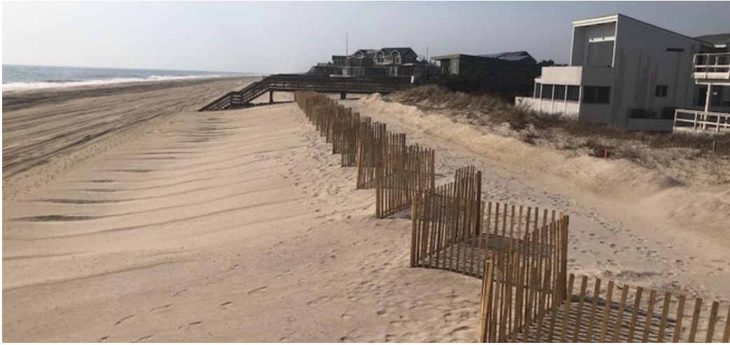
Seaview beachfront after the PL84 repair project (Photo Luke Kaufman)
